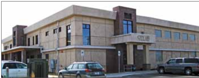
New City Life Building – Almost Completed!
