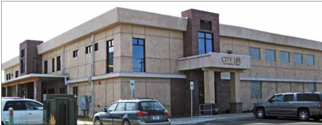
New City Life Building – Almost Completed!
